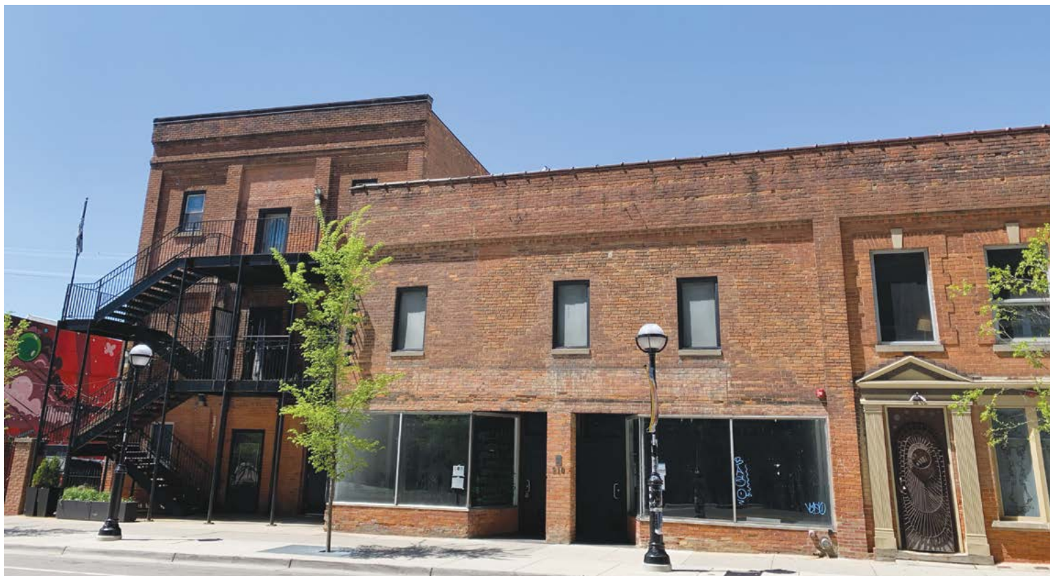
Uplift will be located at 210 First Street in Ann Arbor. Photo: Chris Azzopardi
